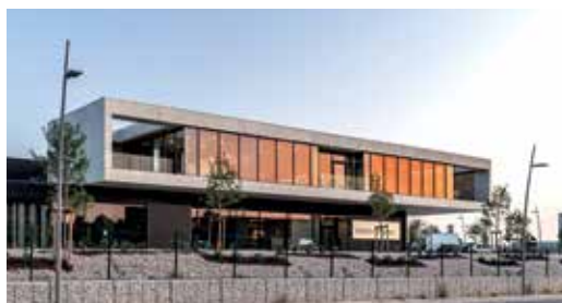
SHOWROOM PORTOVENERE MONTPELLIER, 2021
